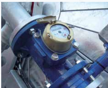
Flanged litre-counter on reel inlet.
